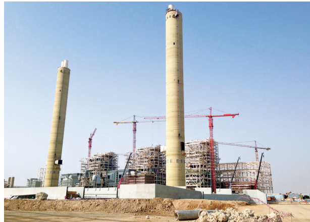
YANBU 2 POWER & WATER PROJECT [Saudi Arabia]
