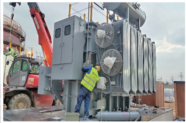
Oil-Transformer Installation
