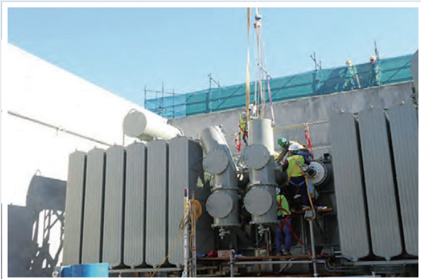
132kV Transformer Erection
