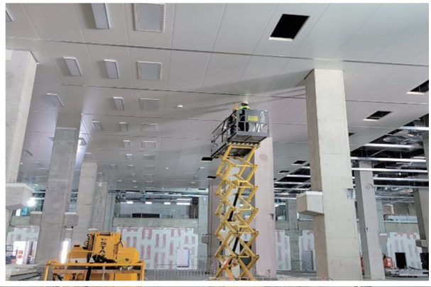
MPB LIGHTING Installation
