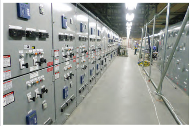
Installation of HVMV SWGR
