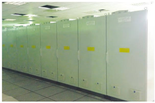
Instrument Panel Installation
