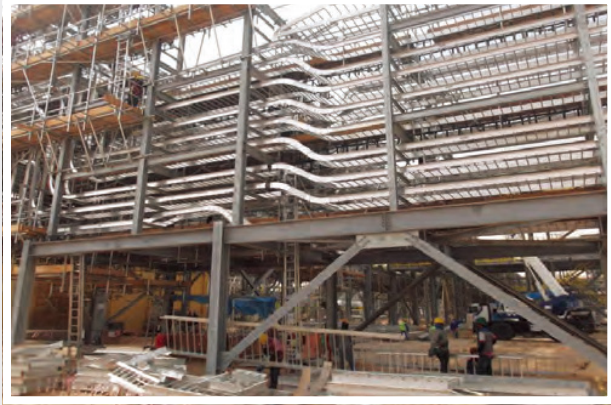
Cable Tray Installation
