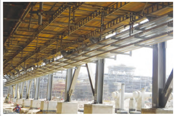
Instrument Cable Tray
