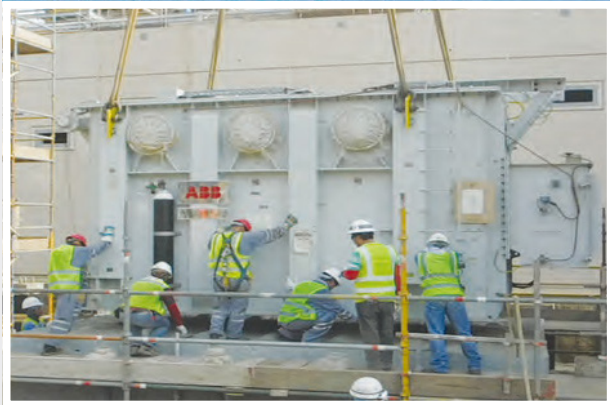
132KV Transformer Erection
