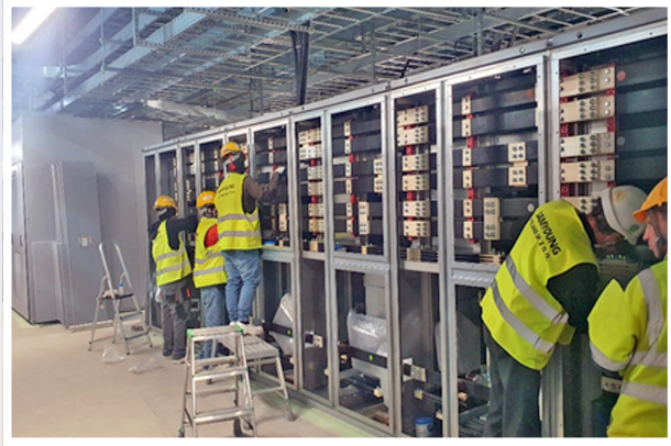
MPB LiBS SWGR Installation
