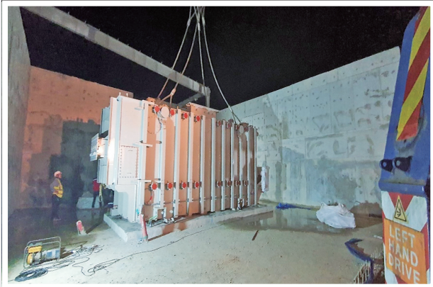
Transformer Erection
