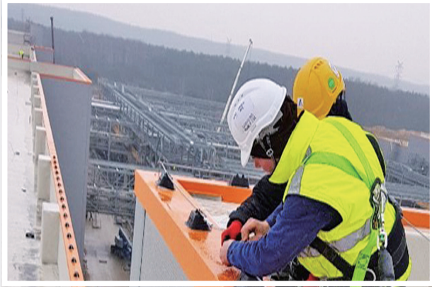
MPB Rooftop lightning wire Installation
