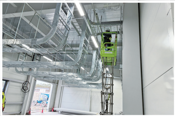
Raceway Installtion
