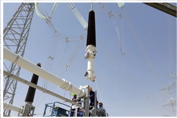
GIB & Gantry Tower
