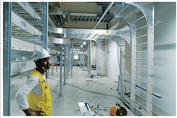
Cable Tray Work
