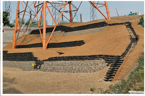
Tower foundation restoration
