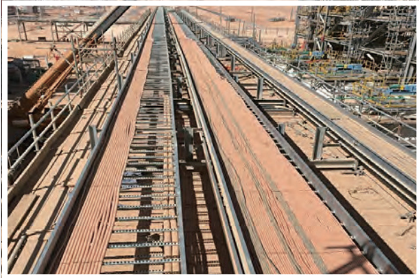
Pipe Rack Cable Pulling
