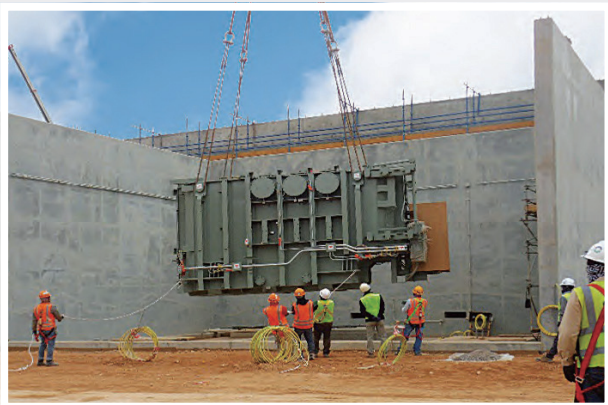
132kV Transformer Rigging
