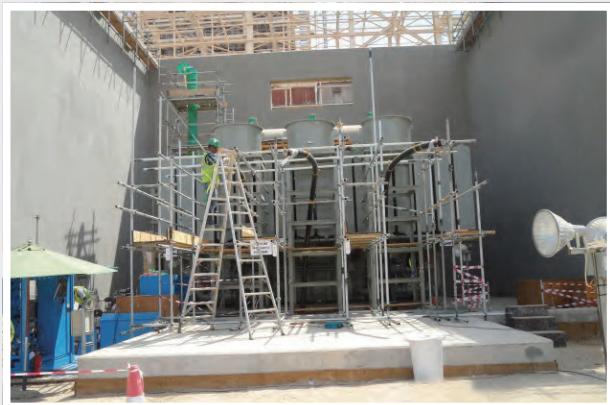
380kV Transformer Erection
