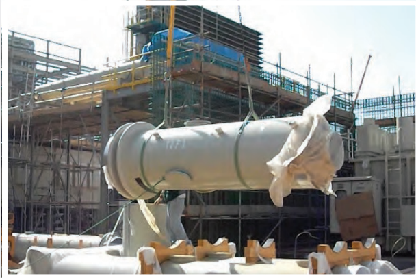
Isolated Phase Bus Duct (IPB) 3PH
