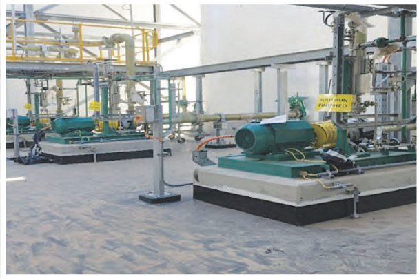
Motor Solo-run Test
