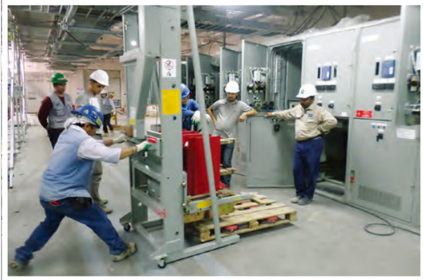
Installation of HV SWGR
