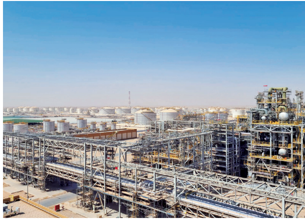
Karbala Refinery Project Area C-1 [Iraq]
