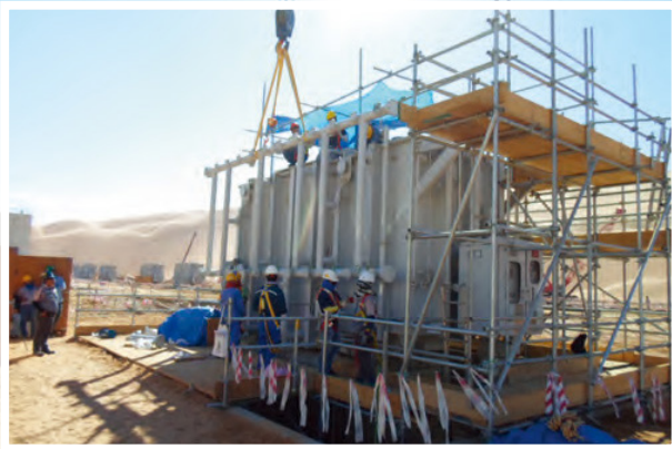
Assembling of Transformer 80MVA
