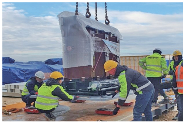
MOLD TR Installation
