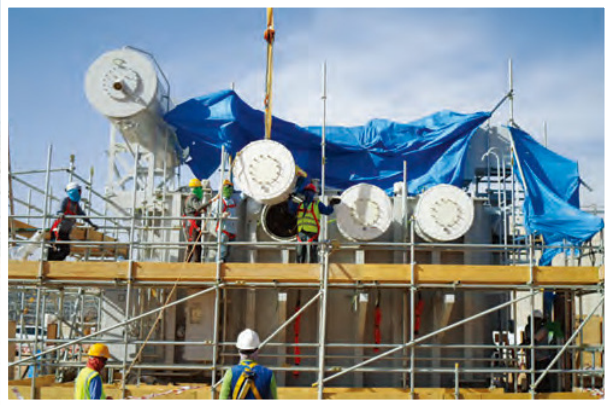
Assembling of Transformer 80-120MVA
