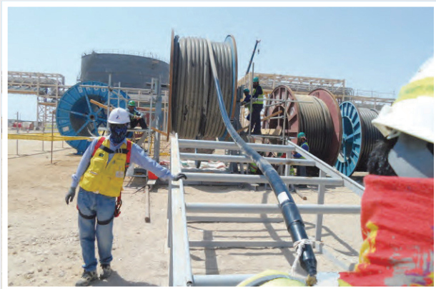
EHV Power Cable Pulling 138KV
