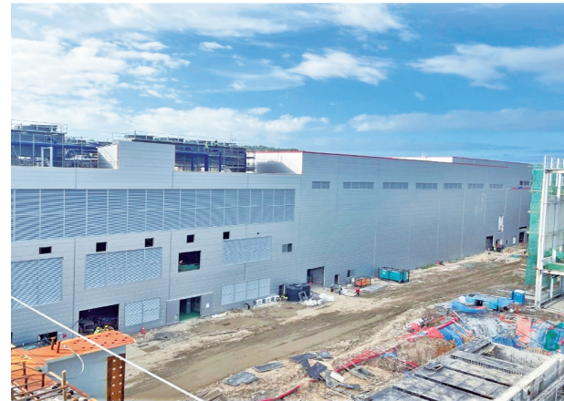
SK Nexilis Malaysia Plant Project [Malaysia]
