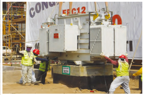
13.8KV Transformer Erection
