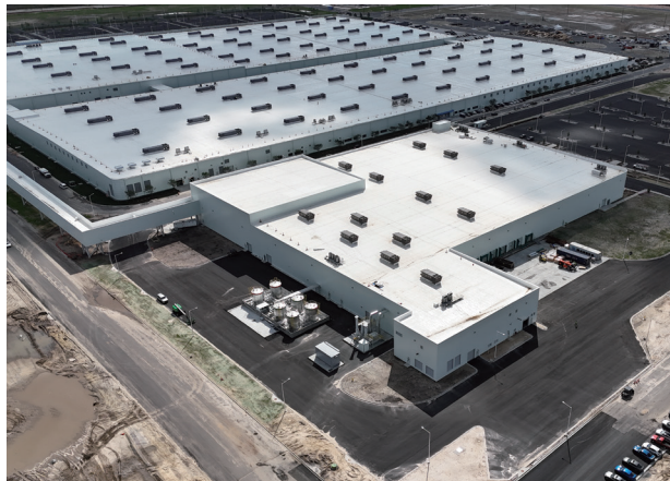
Hyundai Transys Savannah Seat Plant Project [U.S.A]
