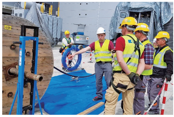
MV Cable Pulling
