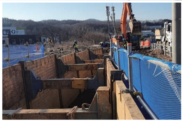
Foundation Rebar Installation
