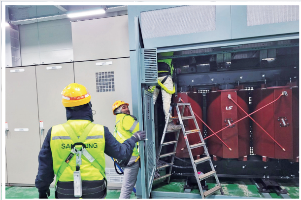
MOLD TR Installation
