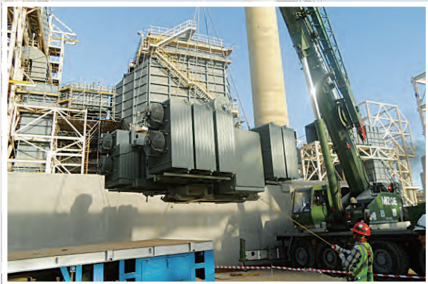
Transformer Rigging
