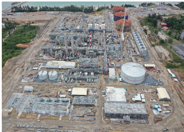
Sarawak PetChem Methanol Project [Malaysia]
