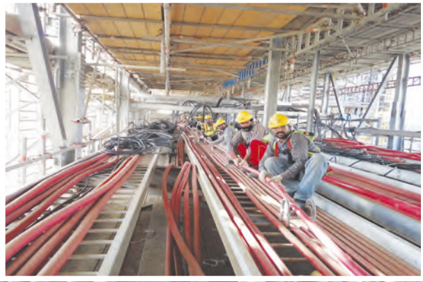
Cable Pulling Work
